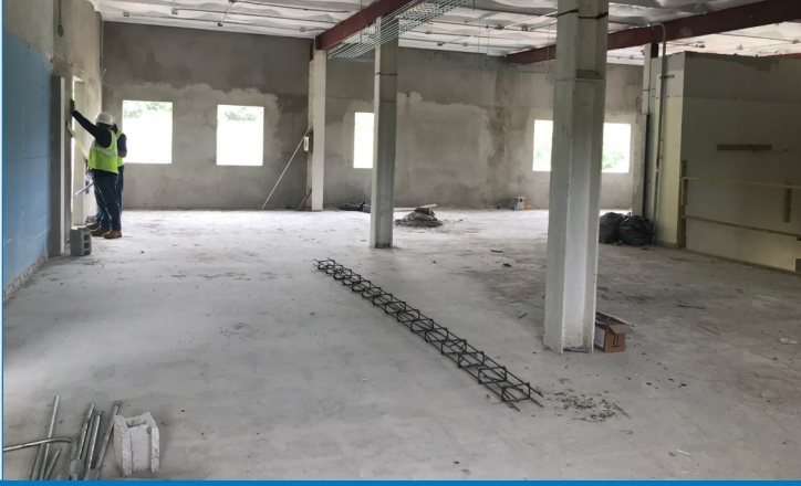
Modifications to the exterior facade have been performed to accommodate new window openings. Masonry work for interior walls, mechanical work, and electrical work are in progress.
