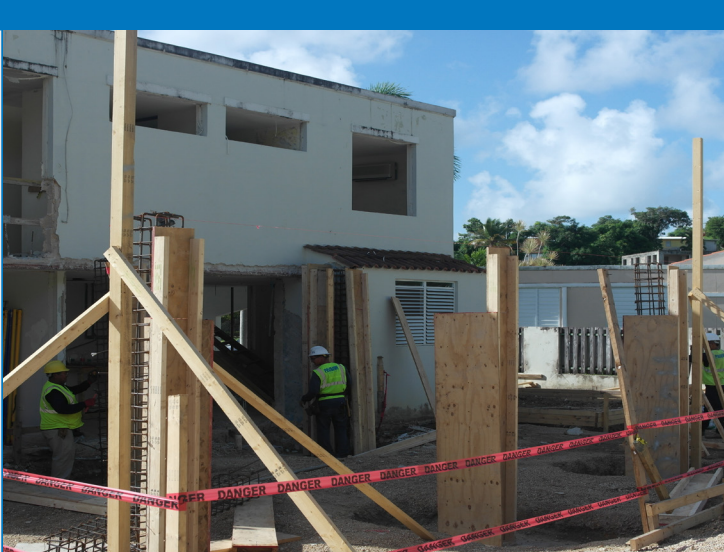
Demolition work has been completed. New foundation work for additions to the structure are in progress.
