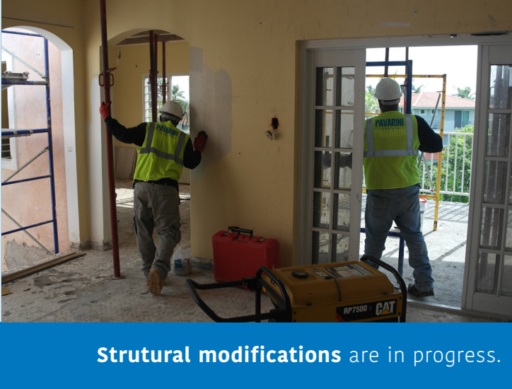
Structural modifications are in progress.
